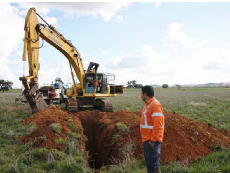
Geotech test pit
