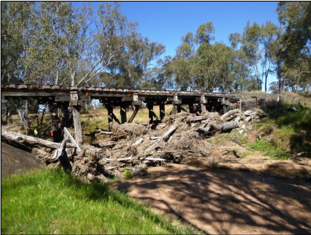
Plate 19: DZP-HS3: Hyandra Rail Bridge with log jam
