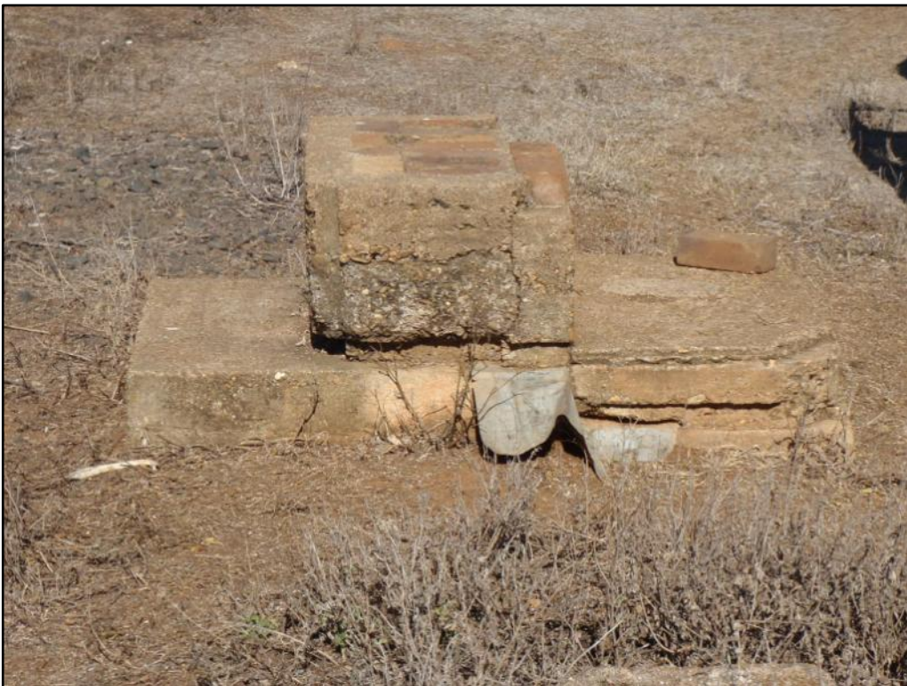
Plate 12: DZP-HS1: Brick and concrete footings.
