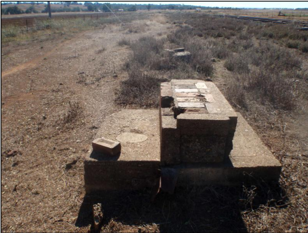
Plate 11: DZP-HS1: brick and concrete footings with second smaller set visible behind them. Rail tracks visible in right background.
