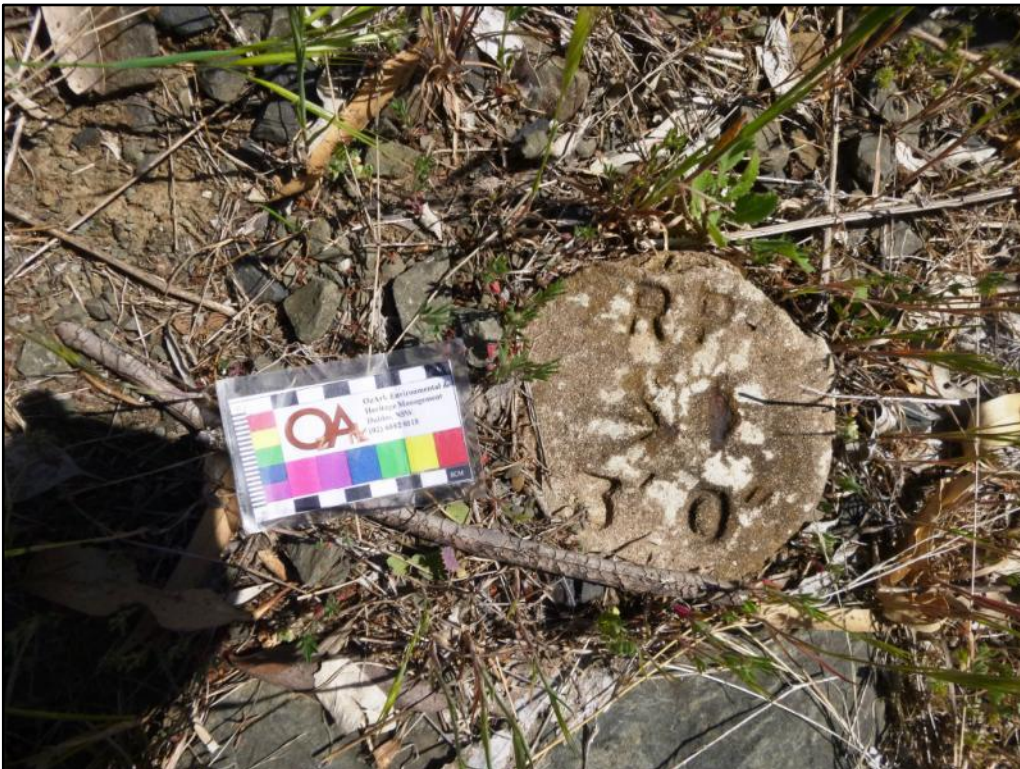
Plate 20: Stamped cement marker at DZP-HS3 Hyandra Rail Bridge
