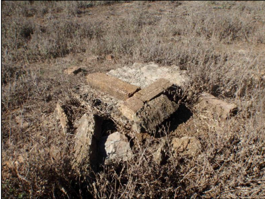
Plate 13: DZP-HS1: smaller set of brick and concrete footings.
