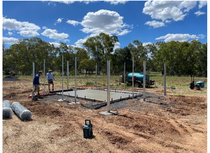
Laying the slab for the monitoring station at Wychitella.
