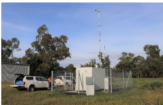
Wychitella environmental monitoring station
