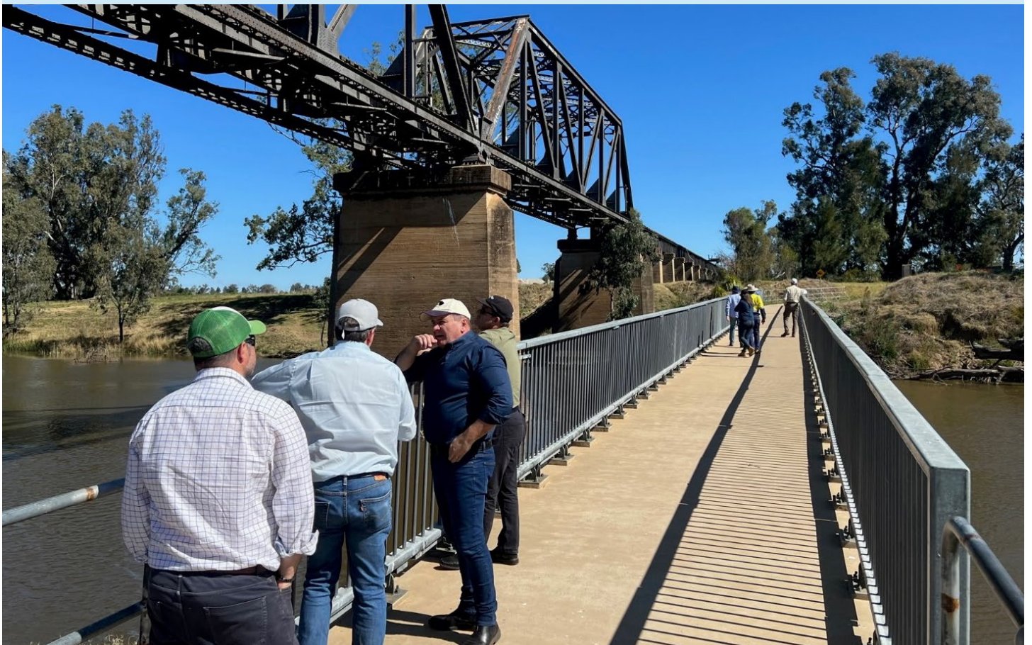
ASM and Bechtel engineers inspecting the Shibble Bridge over the Macquarie River.
